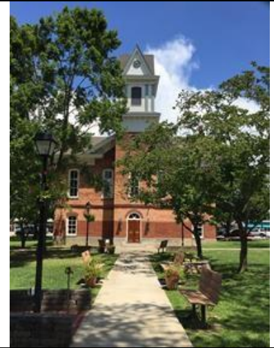
STMS/HHI donated over $16,000 to CCCRA for Historic Courthouse Restoration 2016-2017, completed in 2018 for over $1 million
